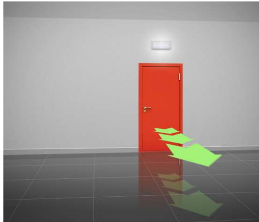
Externally or near every final exit.
