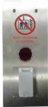
No-entry & Fire-alarm recall key switch (EN81.73)
